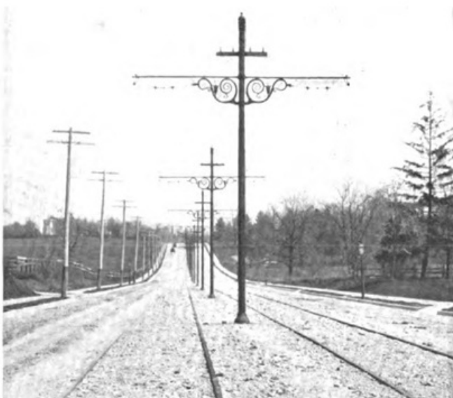
T-RAIL IN CINCINNATI, INTERURBAN RAILWAY & TERMINAL COMPANY
