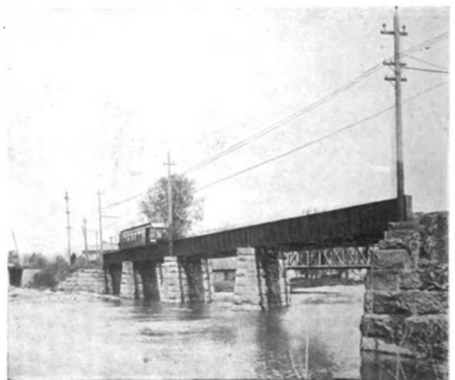
OLENTANGY RIVER BRIDGE, COLUMBUS, DELAWARE & MARION
