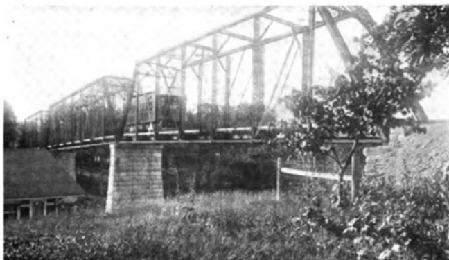
LUDLOW BRIDGE, DAYTON, COVINGTON & PIQUA
