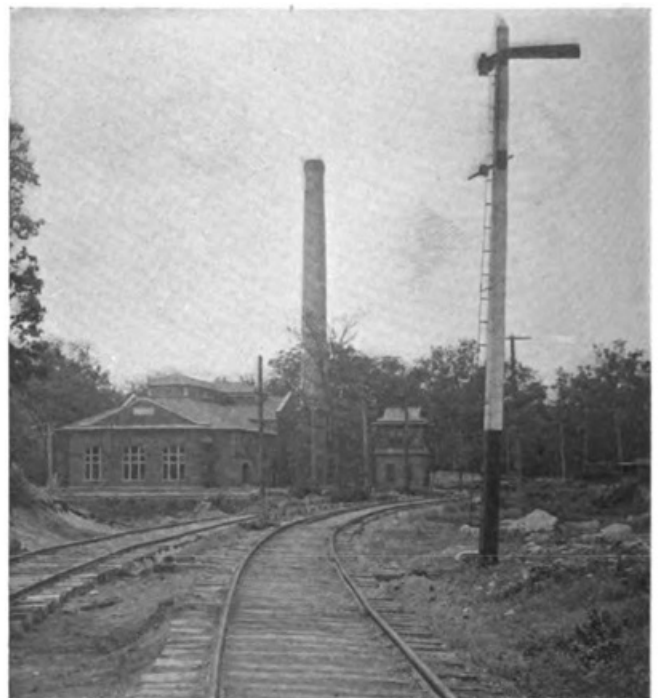
INTERLOCKER AND SEMAPHORE AT RAILROAD CROSSING, SPRINGFIELD, TROY & PIQUA
