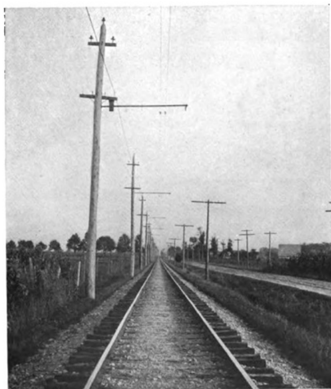
TYPICAL CONSTRUCTION, INDIANAPOLIS, COLUMBUS & SOUTHERN TRACTION
