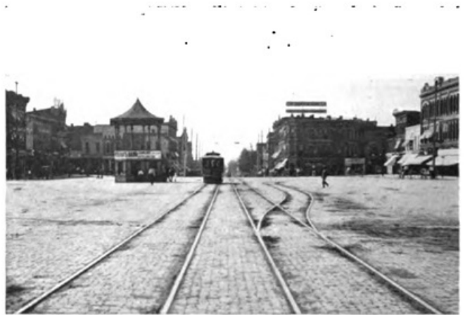
T-RAIL IN LIMA, OHIO, LIMA & TOLEDO TRACTION
