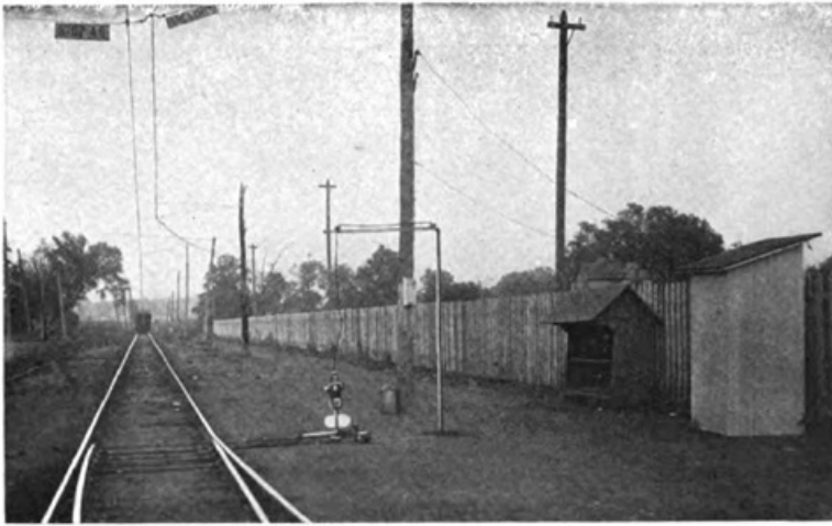
SWITCH LIGHTS, OVERHEAD SIGNS AND TELEPHONE BOOTH TYPICAL TURNOUT, STARK ELECTRIC
