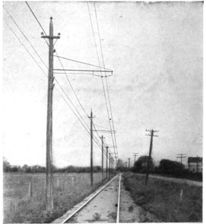
TYPICAL CONSTRUCTION, DAYTON & MUNCIE
