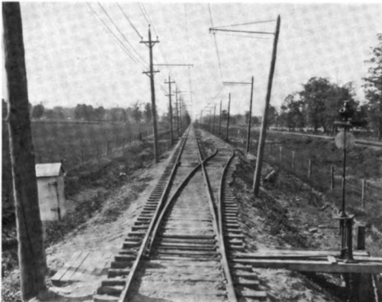
SWITCH STAND AND TELEPHONE BOOTH, TYPICAL TURNOUT, COLUMBUS, DELAWARE & MARION
