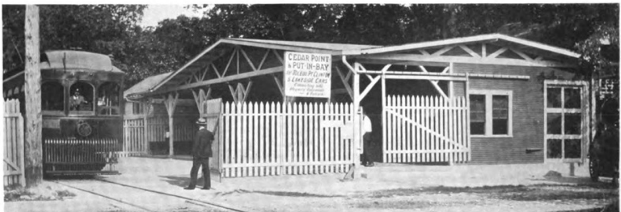
ENCLOSED STATION AT PARK, TOLEDO, PT. CLINTON & LAKESIDE
