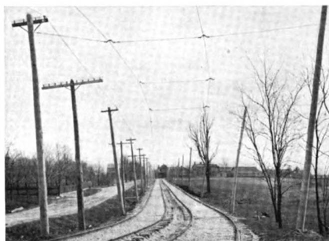
TYPICAL DOUBLE-TRACK CONSTRUCTION, INTERURBAN RAILWAY & TERMINAL COMPANY, CINCINNATI
