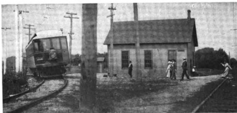
JUNCTION STATION, LAKE SHORE ELECTRIC
