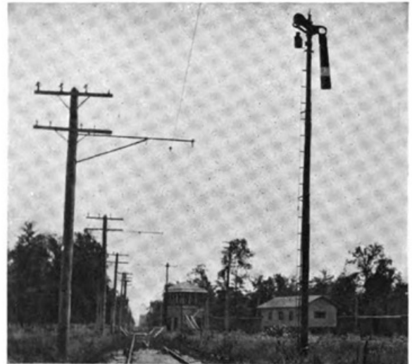
INTERLOCKER AND SEMAPHORE AT RAILROAD CROSSING, TOLEDO & WESTERN
