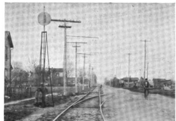
SWITCH STAND AT TURNOUTS, COLUMBUS, LONDON & SPRINGFIELD
