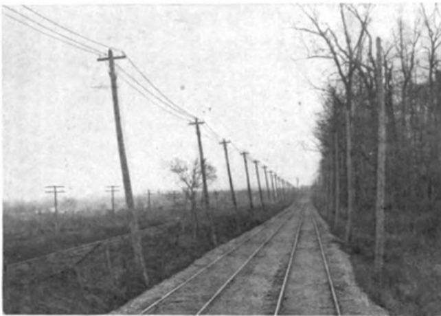
DOUBLE-TRACK CONSTRUCTION, DAYTON & TROY
