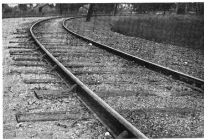
CURVE CONSTRUCTION, INDIANA UNION TRACTION
